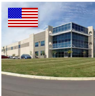
Made in the USA at Tresco's manufacturing facility in Louisville, KY
